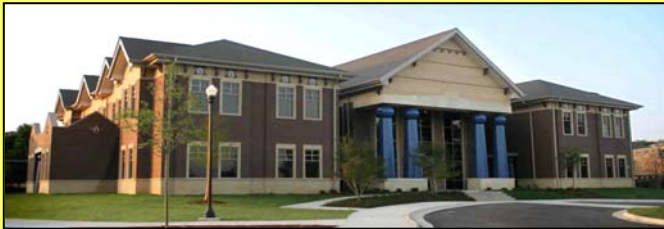
NCAC Community Services Building
